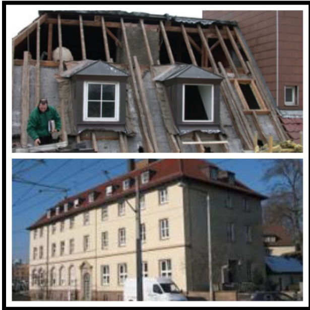
Figure (4-6): Nursing home, before and after (BRITA in PuBs, 2008)
