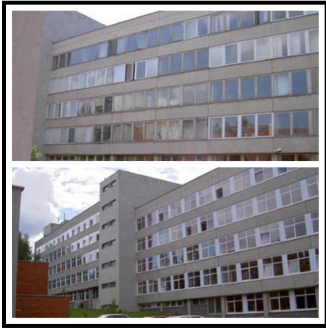
Figure (4-7): Technical University, before and after (BRITA in PuBs, 2008)
