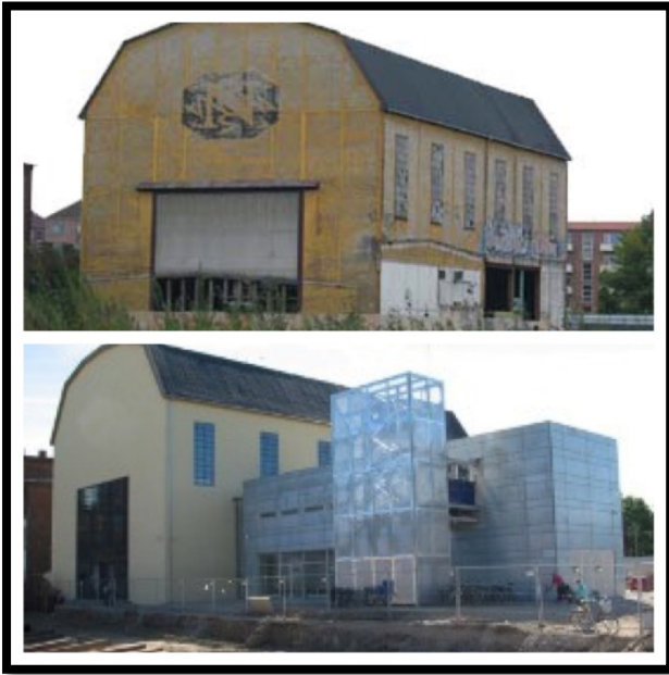
Figure (4-5): Cultural centre, before and after (BRITA in PuBs, 2008)
